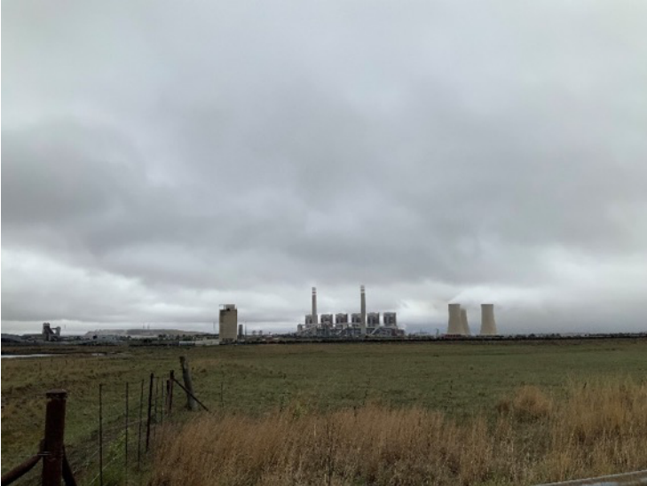
Figure 7: Majuba Power Station
